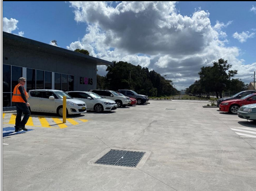
PHOTO 6 – COMPLETED CARPARK AND STORMWATER DRAINAGE PIT
